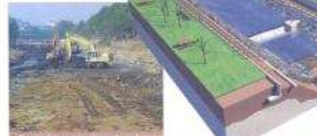
The dredging operation gets underway.
