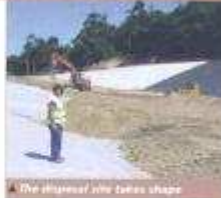
The disposal site takes shape.
